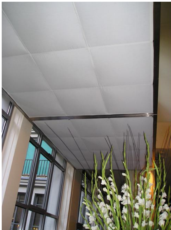
Figure 19: “down flow” cloth fastened with Velcro in segments of 0.6 by 0.6 metres.
